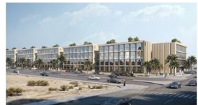
Asala Residence Mohamed Al Habib Real Estate Company Riyadh, Saudi Arabia
